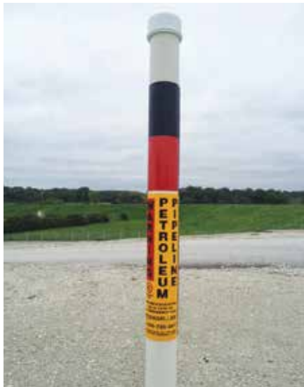
Our pipeline markers can be typically identified by the black and red bands at the top.
